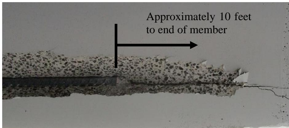
**Figure 2**– Termination of bar in failed double tee
