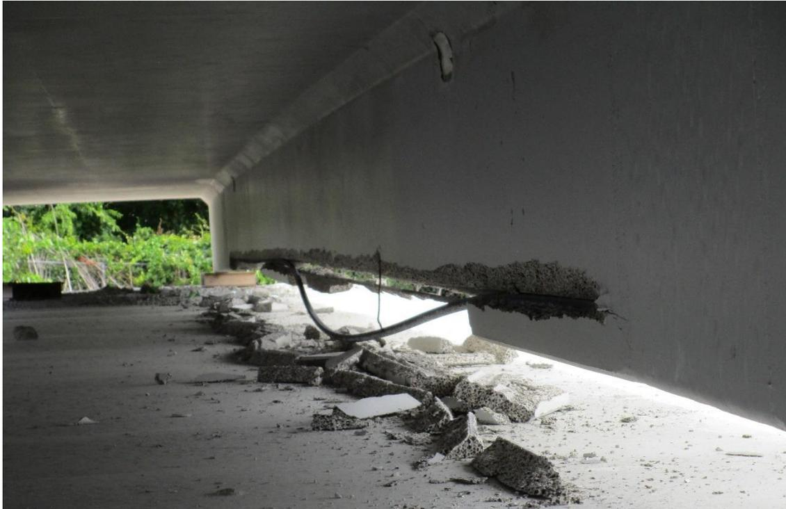
**Figure 1**– Failure of double-tee stem due to creep-rupture
