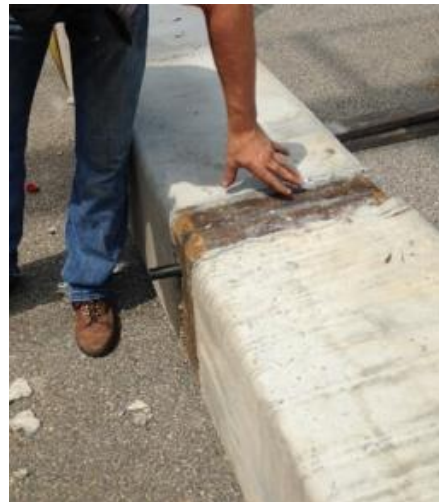
122 123 Fig. 4 – Splice connection during alignment (left) and installation of locking pins (right) 124
