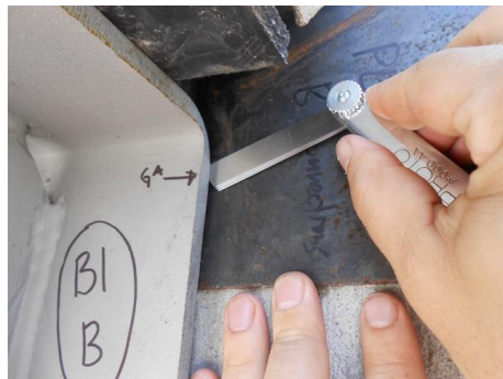
Figure 7 - Measuring gap behind gusset plate
