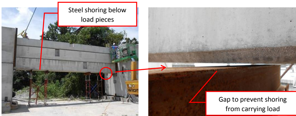
Figure 4 - Shoring below precast member during testing
